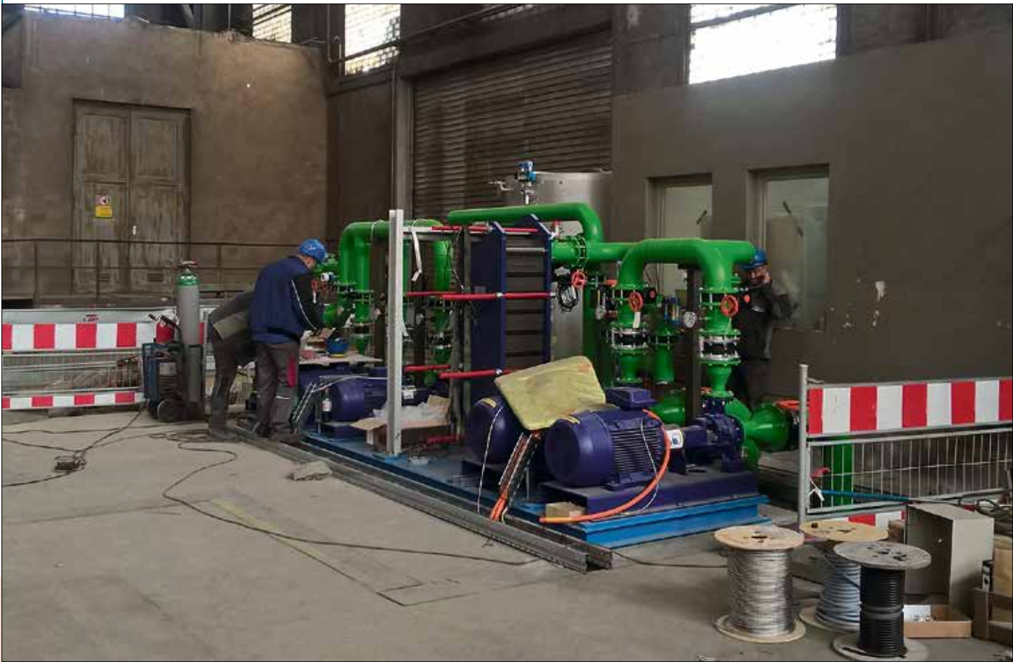
Liebscher specialists install the new return-cooling system.
